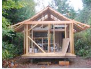
Building a shed, Marrowstone Island Homestead
